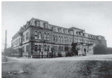
Tokyo Higher Technical School Main Building in Kuramae
